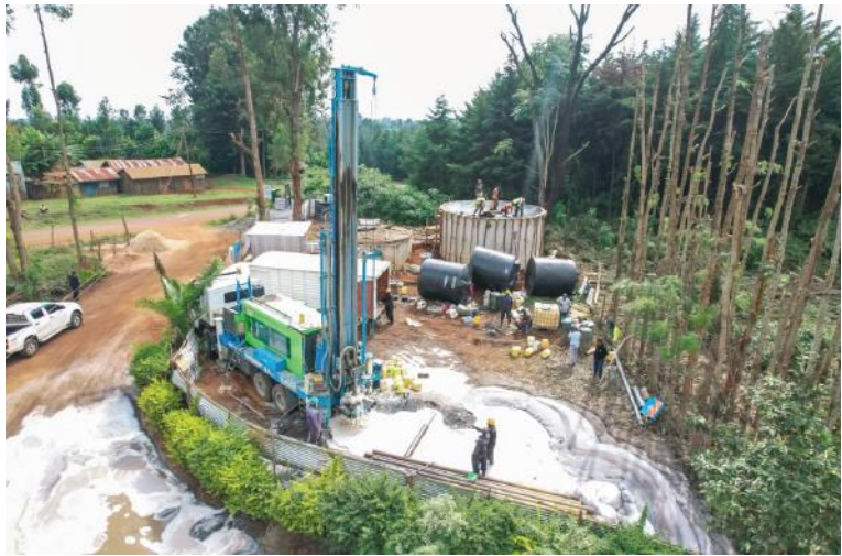
Jiinue Rupingazi Water project borehole under construction
