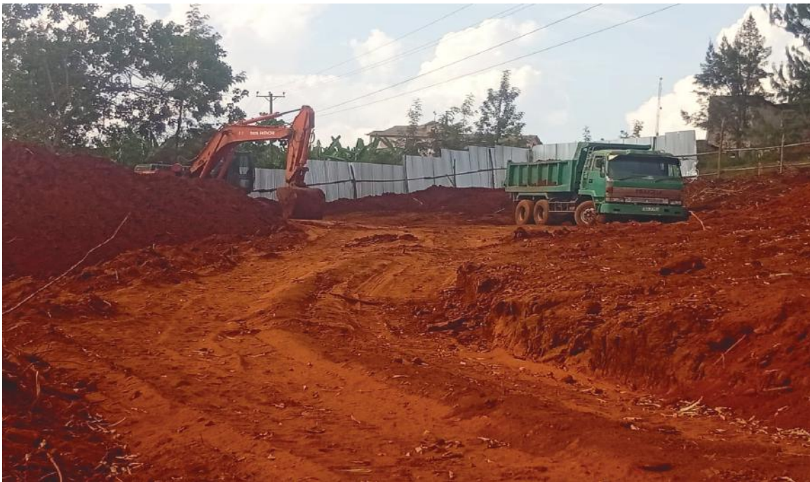
A section of the ongoing affordable housing project in Gatundu South Kiambu County.
