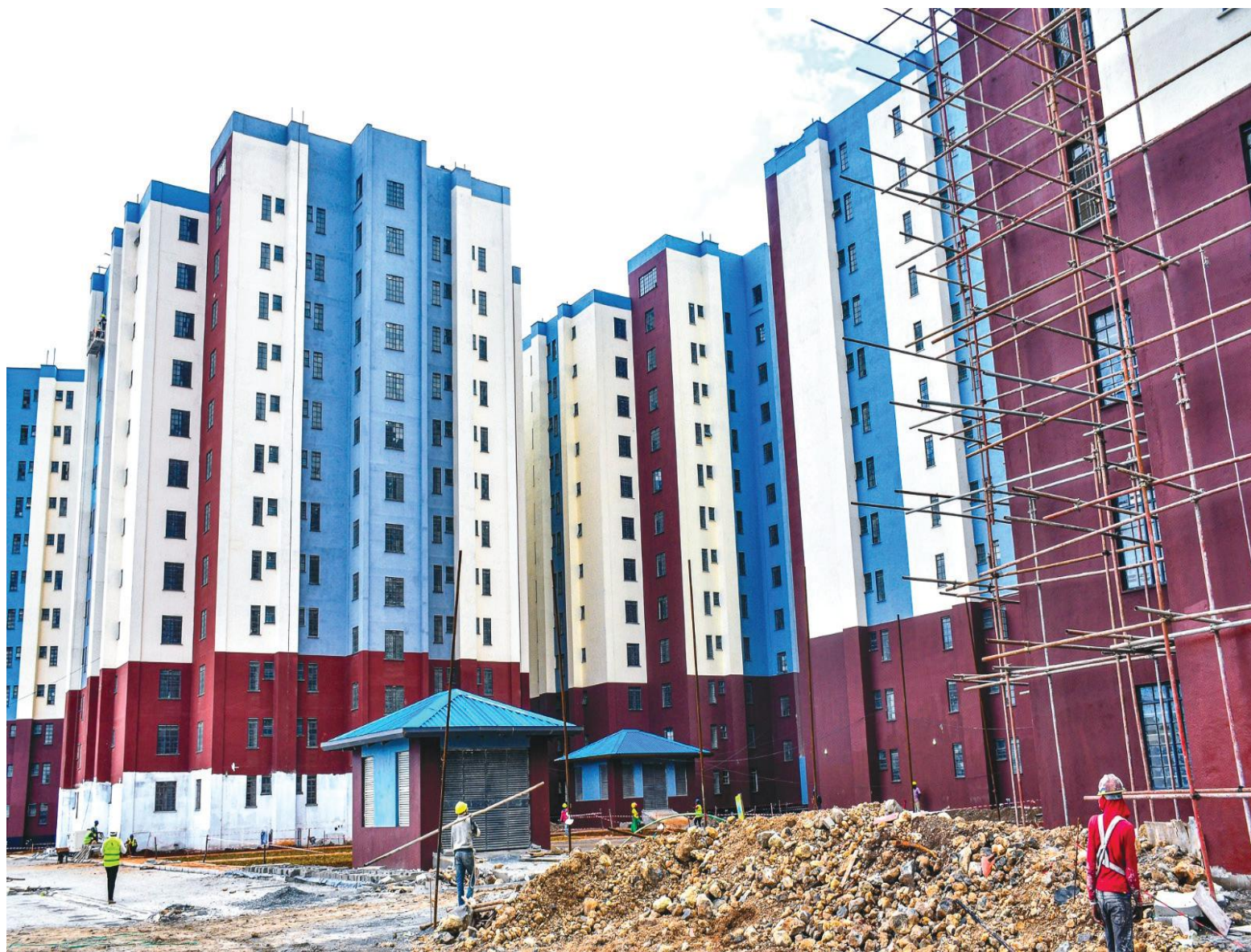
The Mukuru social housing project in Nairobi.
