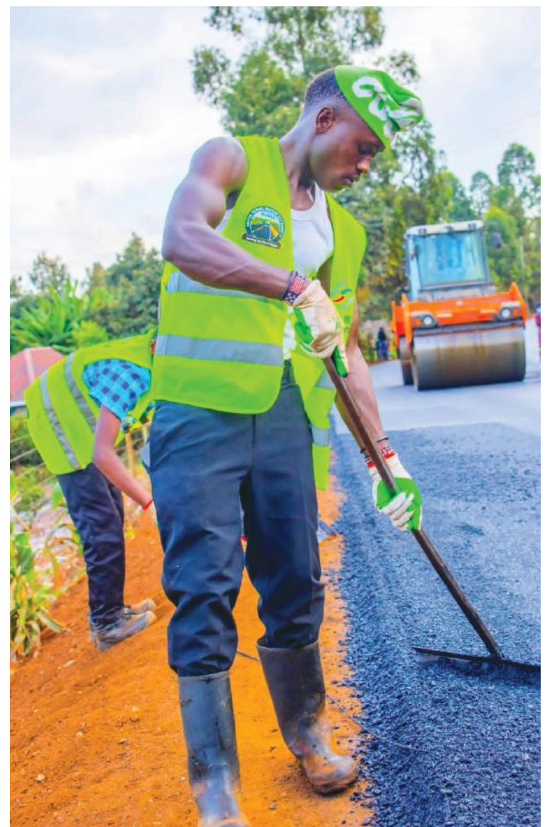
Tarmacking of Kaiyaba-Muchatha road in Kanunga location
